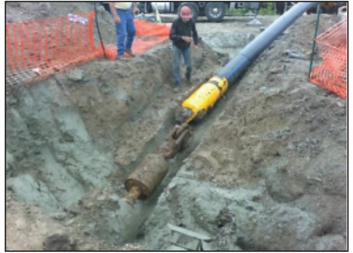
Figure 10 – Pipe Pullback
