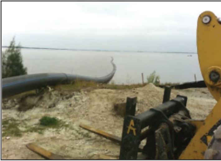
Figure 9 – HDPE Fused Pipe String-out
